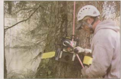
ALEX PAJUNAS — The Daily Astorian Mike Newby, removes any slack from the rope running through the Good Rigging Control System strapped onto the trunk of a Sitka spruce tree. The system allows for the removal of problem trees without having a person in the tree cutting. Instead pieces could be cut from the bottom.
